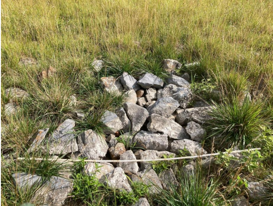
Figure 2.5: Filled sinkhole near the artificial pond.
