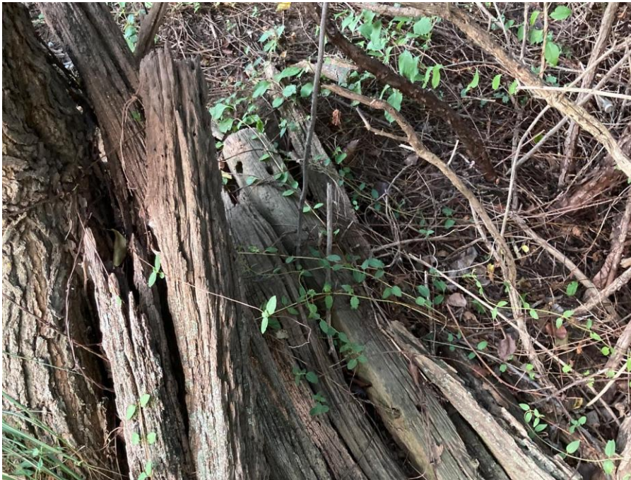
Figure 2.6: Pile of demolished split rail fence at a former property boundary within the project area.
